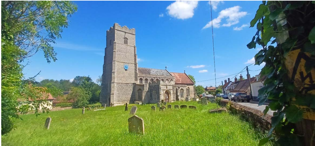
Figure 6: St Mary's Church, Badwell Ash.
