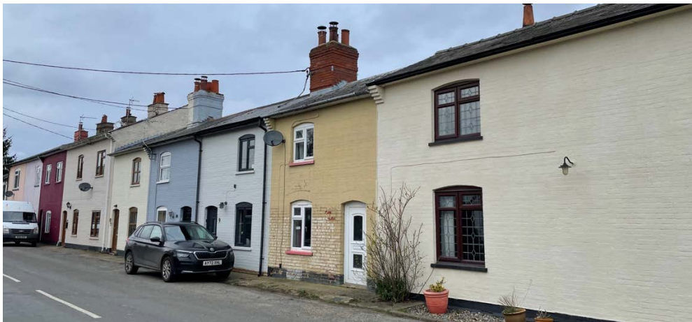
Figure 8: Long Thurlow Road, Long Thurlow.
