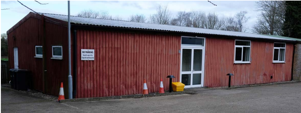
Figure 34: Badwell Ash Village Hall.
