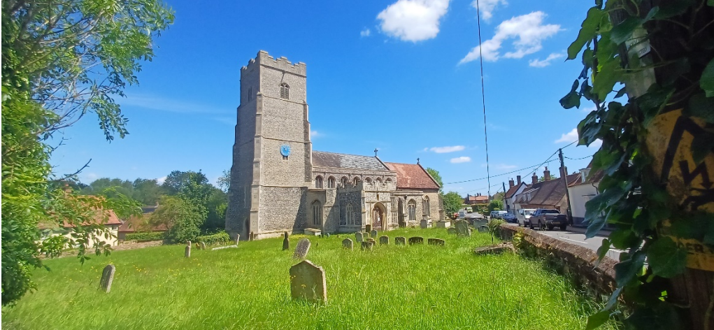
Figure 6: St Mary's Church, Badwell Ash.
