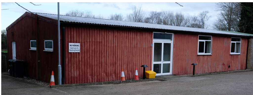
Figure 34: Badwell Ash Village Hall.
